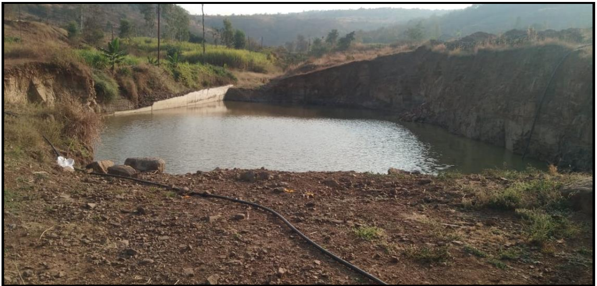
Water Harvesting site : Check dam constructed at Wagjai Site of 60,00000 Liter Capacity.
