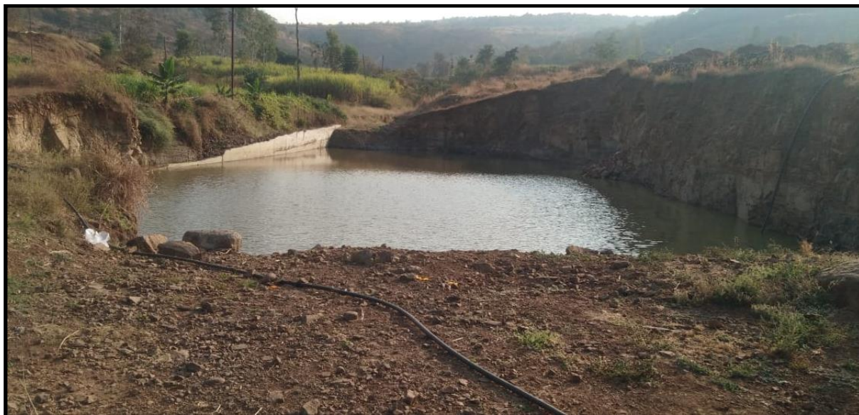
Water Harvesting site : Check dam constructed at Wagjai Site of 60,00000 Liter Capacity.(Photo- 2)
