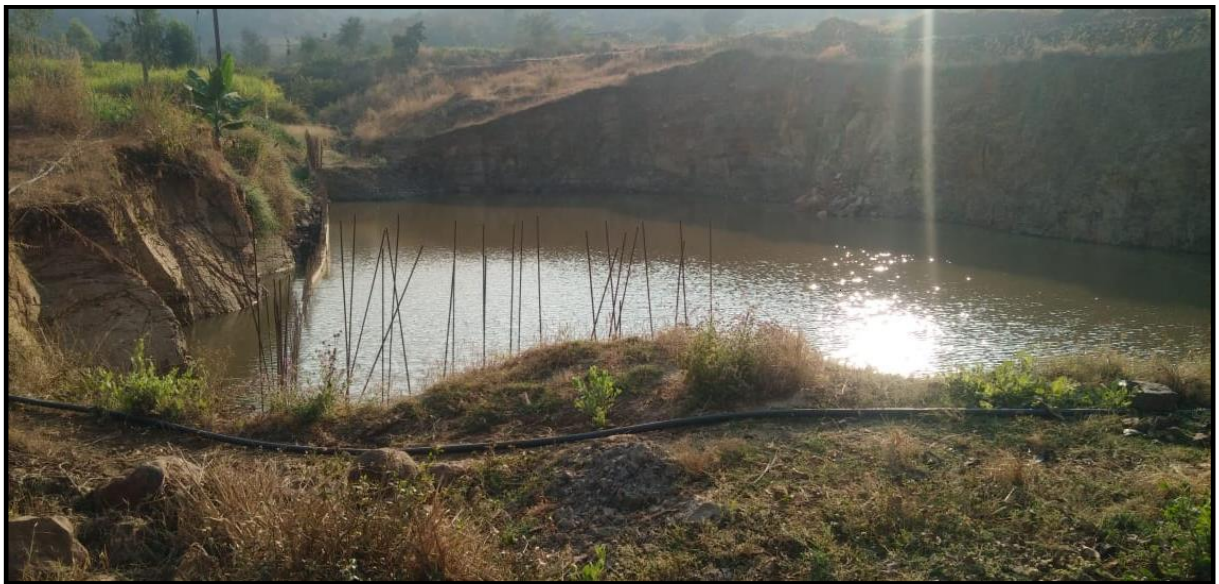
Water Harvesting site : Check dam constructed at Wagjai Site of 60,00000 Liter Capacity.(Photo- 1)
